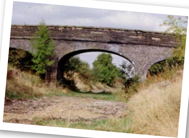
Bridge No.488 with its parapet of dressed stone. PHOTO: JOHN QUICK
